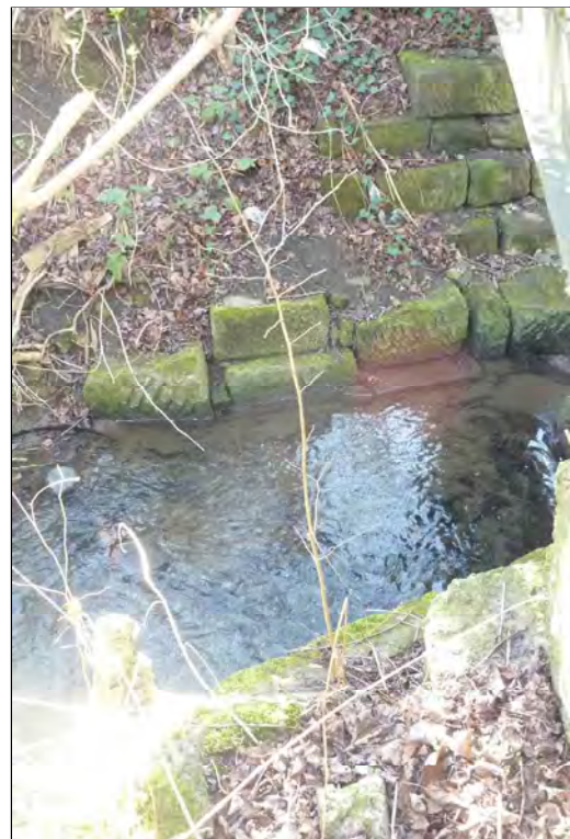
Stone revetment of leat by Rainton footbridge
