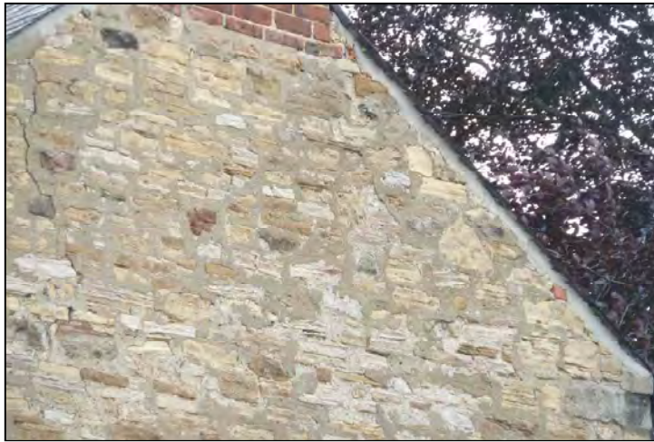
Traces of an earlier, steeper roof line for thatched roof
