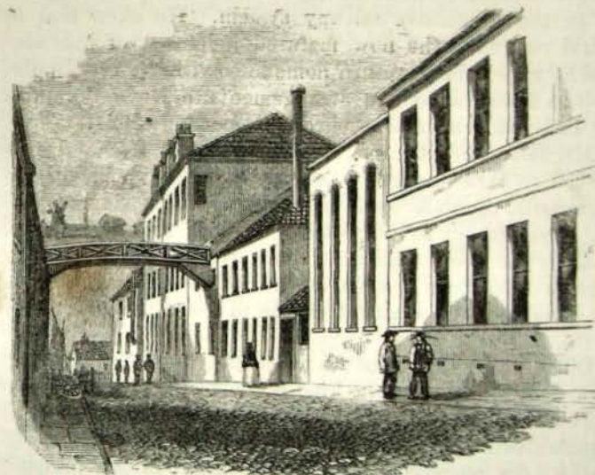
Forth Street Works, Newcastle.
