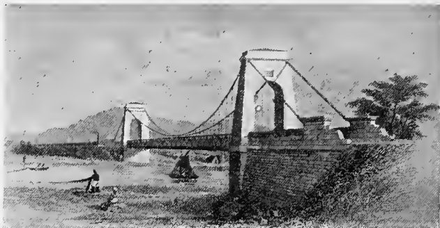
END VIEW OF THE FIRST RAILWAY SUSPENSION BRIDGE IN THE WORLD.
