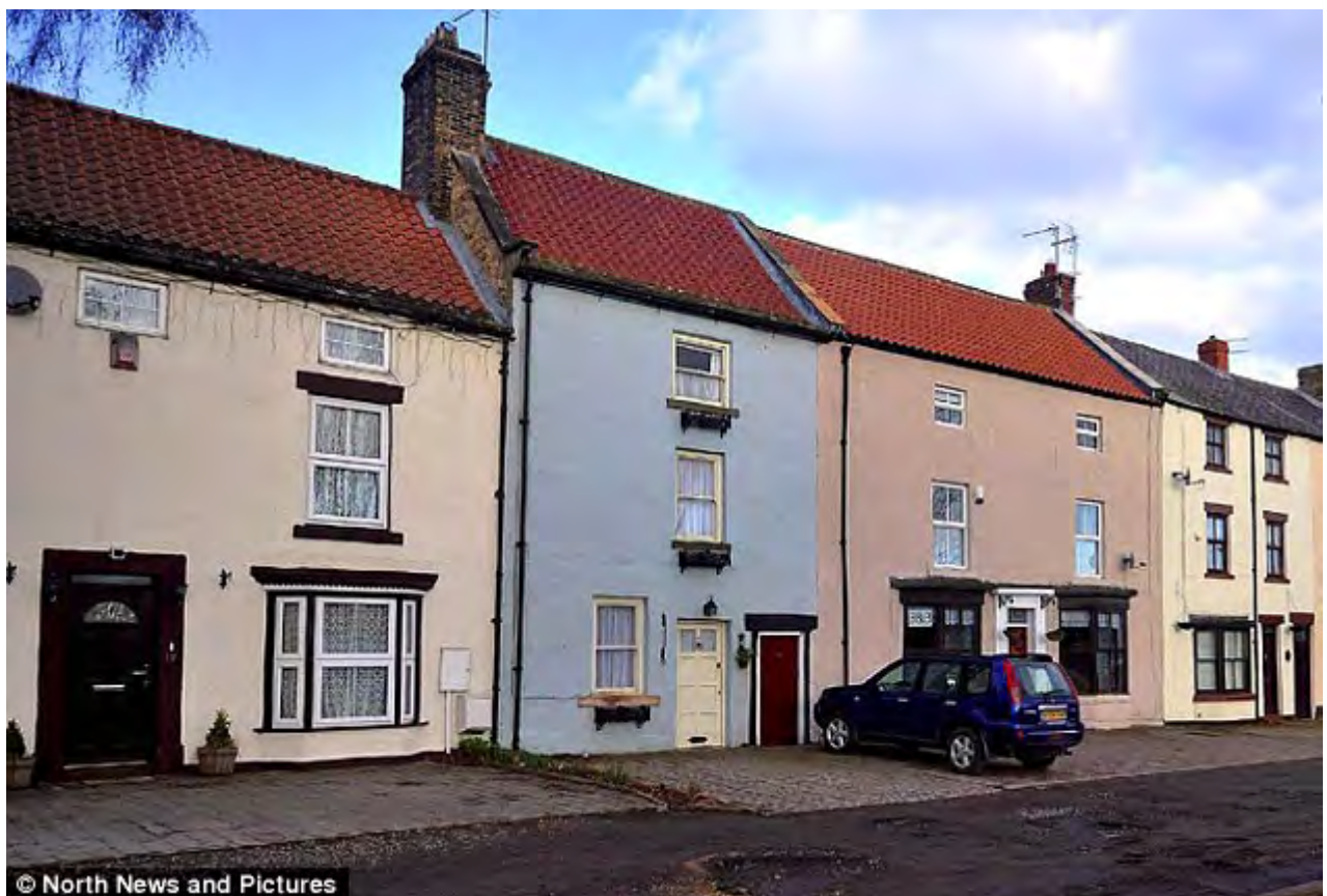
The property as it is today, painted blue, has changed very little from what it looked like in 1873
