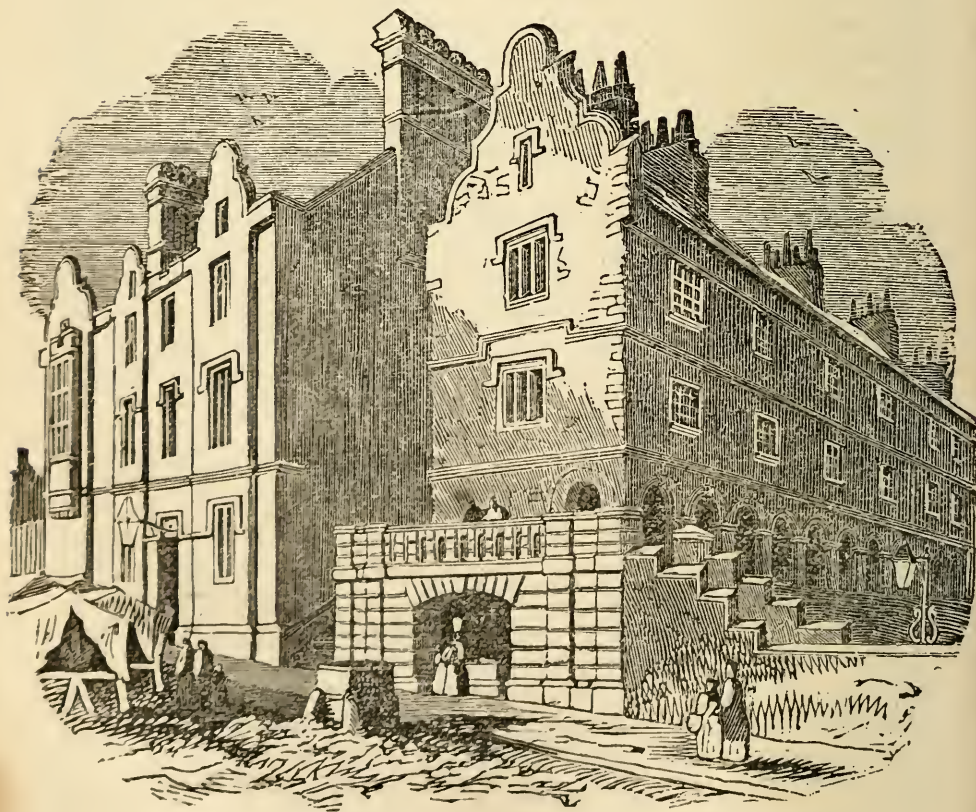
POLICE STATION, MANORS, AND FREEMEN'S HOSPITAL.
