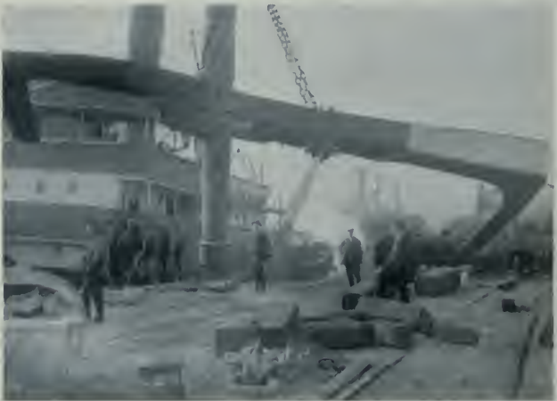
Stern frame of the Britannic being loaded at West Hartlepool
