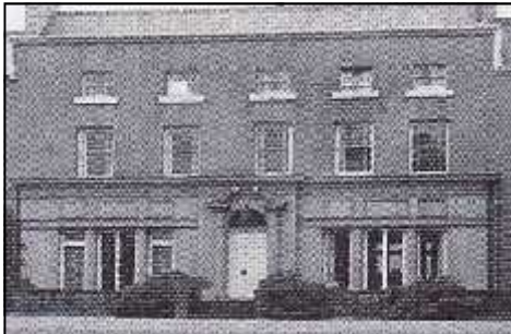
This aspect shows the original Georgian Hall incorporated in the Victorian additions together with changes to the fascia
