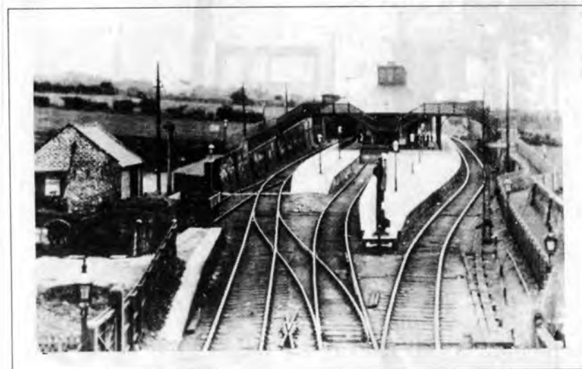
Leamside Station in the early 1900's
