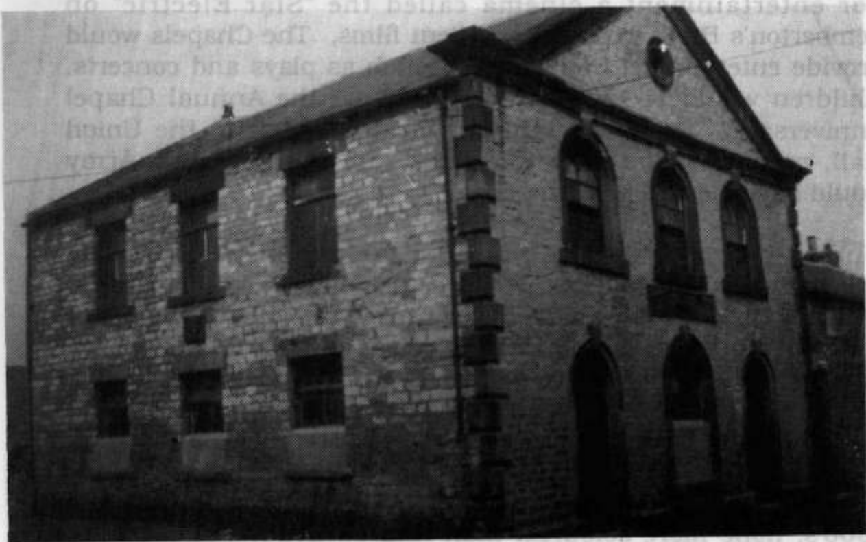
The Primitive Methodist Chapel built 1869 demolished 1977
