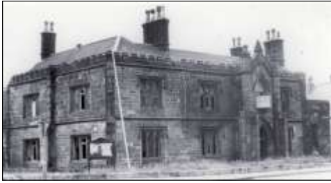
The Infirmary, Tempest Place built 1844 with money from Frances Anne. It was demolished in 1969
