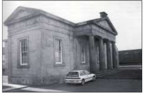
Literary institute, built in the middle years of the 19th century. It is now used as flats for aged miners.
