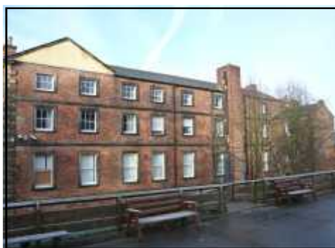
Rear of Building
