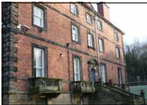
South side entrance Elemore Hall
