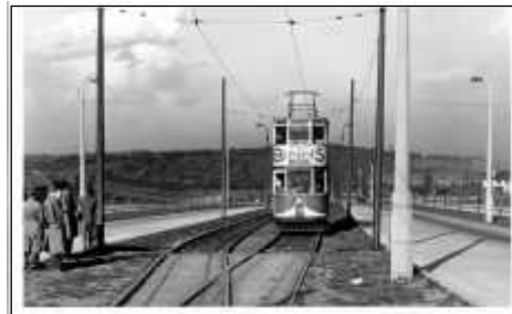
Last section of tramway to be built to Thorney Close in 1949. It was also the first to have a dedicated tram track rather than use the existing road system.
