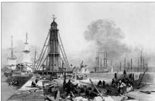
Construction of the early North Pier lighthouse
