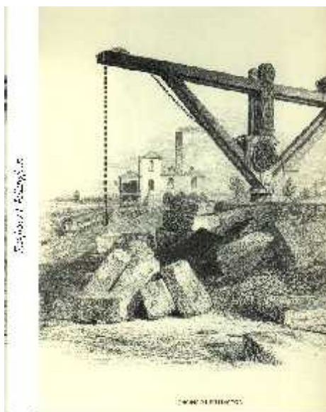
Pittington Engine—drawing by Hair 1844. Note the drums on the side of the building and the strange little carriages for passengers. View from station platform.
